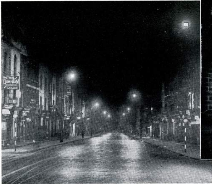
Park Street, St. Pancras, lighted by 400w. Sieray "H" type Lamps in Regent-Sieray Lanterns.
