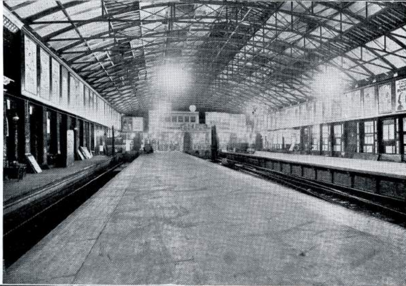
Fenchurch Street Railway Station lighted by a combination of 250w. Sieray 'H' and Tungsten Filament Lamps in Preston-Sieray Lanterns.
