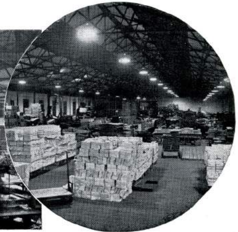
Printing Works illuminated by 400w. Sieray 'W' type Lamps.
