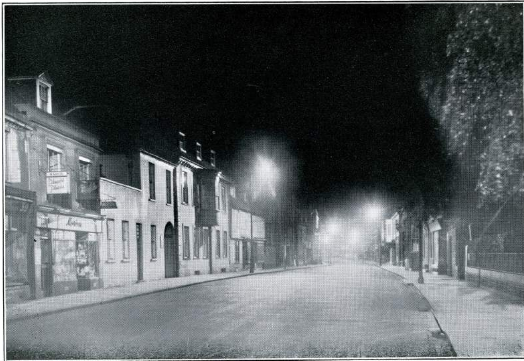
North Street, Chichester, lighted with Siemens 400 watt Sieray 'H' type lamps.
