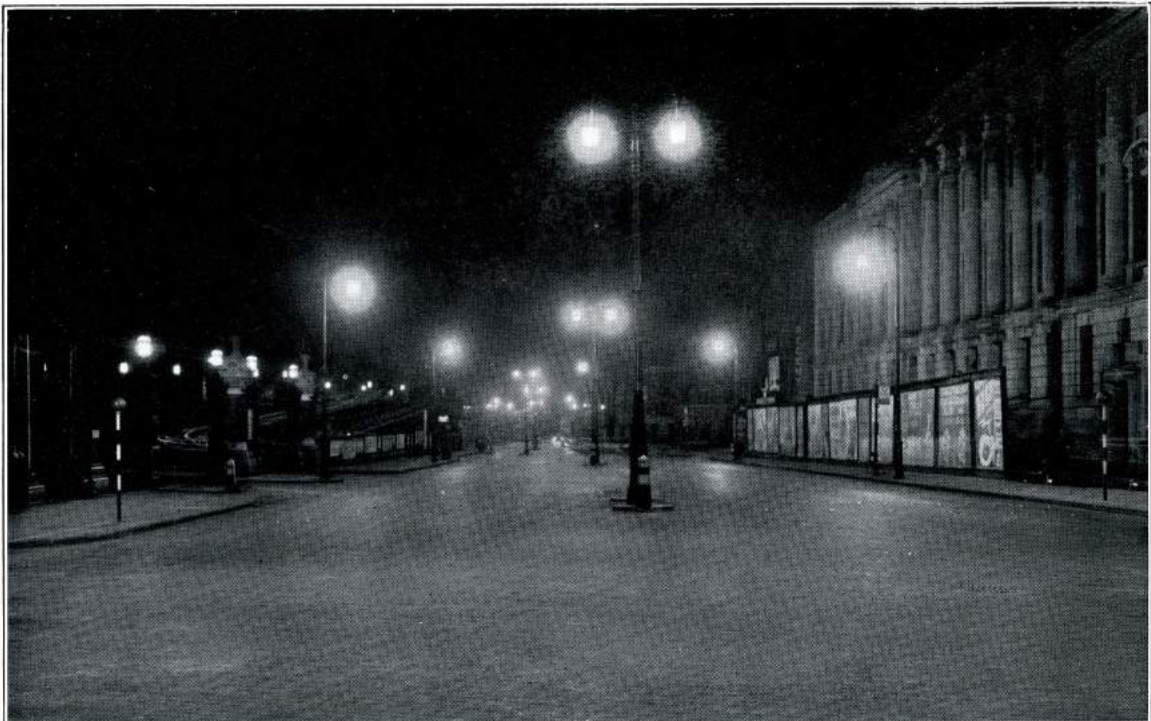
Euston Road lighted by 400 watt Sieray "H" type lamps in Regent-Sieray Lanterns.
