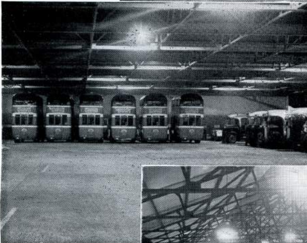
West Riding Auto Company's Garage, Wakefield, lighted by "Sieray-Dual" Lamps in Dispersive Reflectors.
